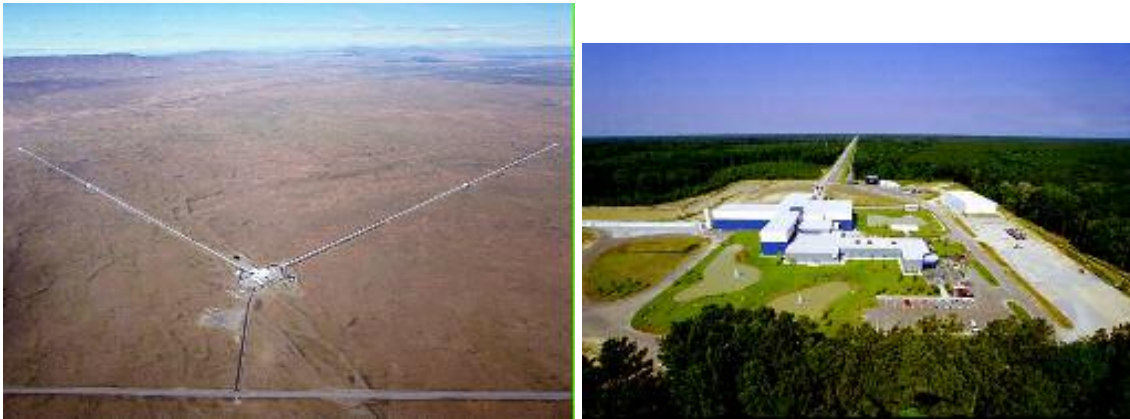
Figure 3: These pictures are of the LIGO interferometers themselves. On the left is the Hanford Observatory which houses a 4 km interferometer, and a 2 km interferometer. On the right is the Livingston Observatory, which has a 4 km interferometer. [ http://www.ligo.caltech.edu ]
