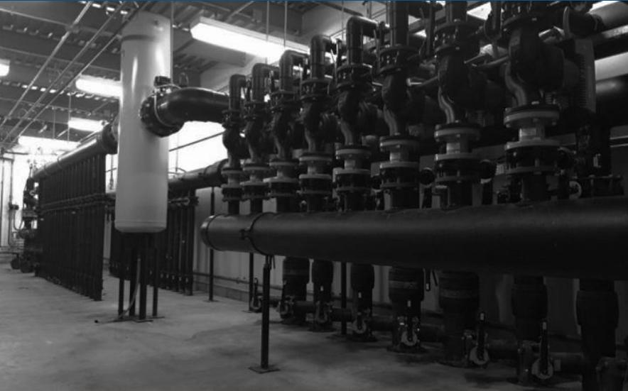
Skidmore installed its first geothermal heating system in 2007 in conjunction with the construction of new student housing. Skidmore has since completed two additional geothermal projects that supply heat to several other buildings on campus. Together, these systems supply 40 percent of the campuses' heat. The boreholes were drilled to between 400 and 500 feet and cost the college approximately 1.4 million.
